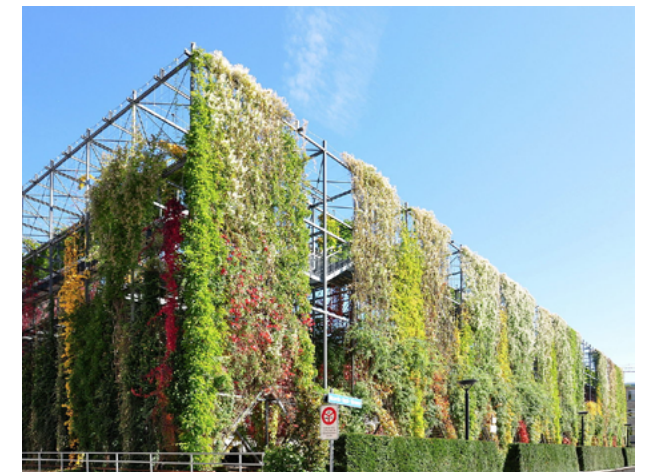
Groene gevel MFO Park in Zürich
